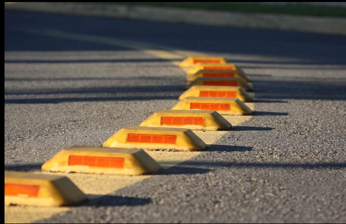
Raised pavement marker
